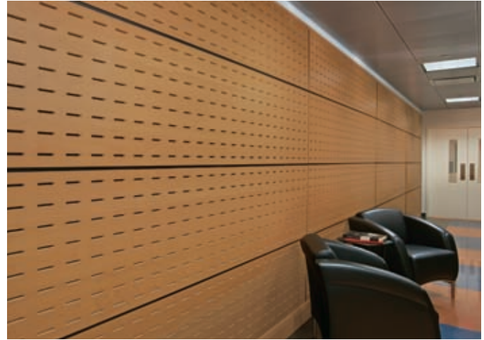
WoodWorks Wall System 2' x 9' panels with W6 perforation in Natural Variations Light Cherry; Finish Molding in Natural Variations Light Cherry
