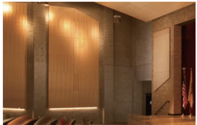
WoodWorks Wall panels on Z-clips with W2 perforation in Custom Maple
