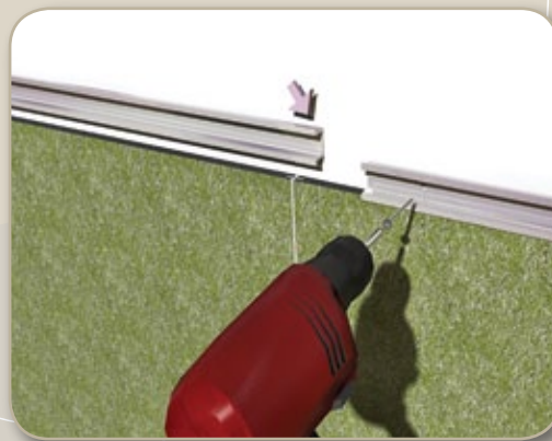
3. Secure the Panels and add horizontal detail with your choice of Reveal options
