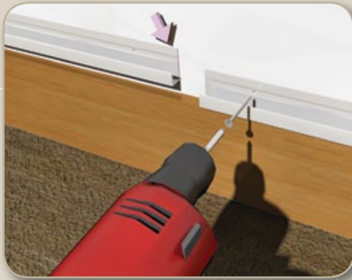
1. Attach the CP280 Edge at bottom of installation, along with all Perimeter Trim
